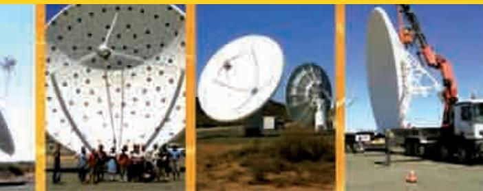
in the Northern Cape. The development of seven dishes, called KAT 7, has already been completed. KAT 7 is a prototype that will be used to test all of the telescope systems – the antennas, the receiver systems and the complex software and computing systems.
