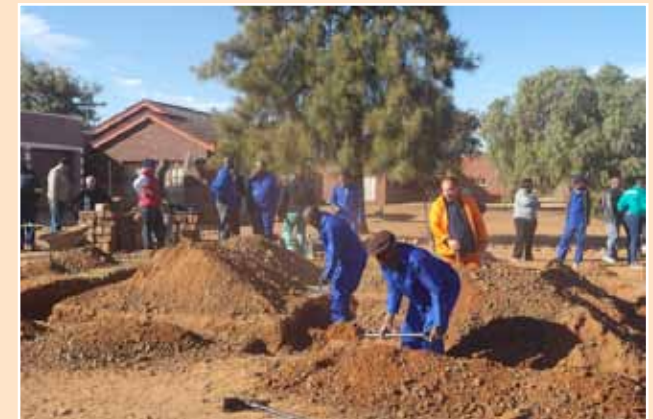
Municipal officials working hard during the sod-turning event in Mapoteng.
