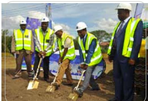
MOVING EARTH: MEC for Health with officials from the Eastern Cape Department of Health and the Coega Development Corporation break ground on the Sipetu District Hospital project.
