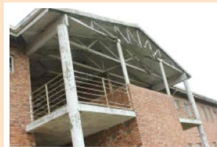
**Part of the roof of the first-floor balcony falling apart.**
