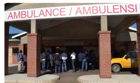
The emergency entrance to the impressive facility.
