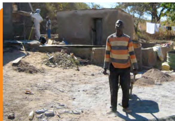
At work, volunteers building the house for a needy family.
