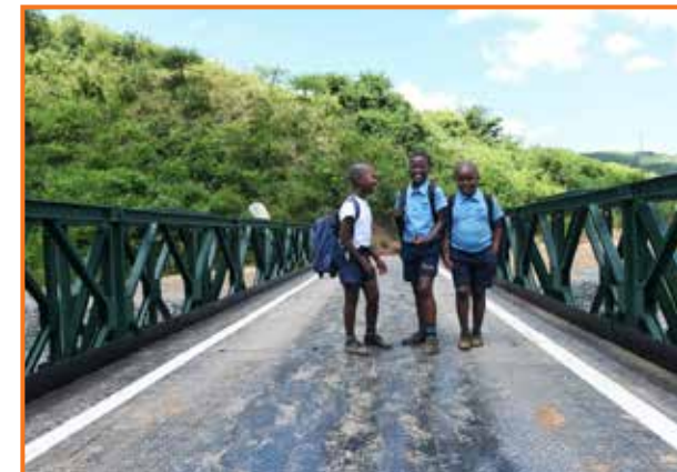
Jubilant school children crossing over the newly built bridge.
