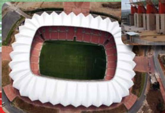
Nelson Mandela Bay Stadium, Port Elizabeth
