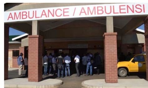
The emergency entrance to the impressive facility.
