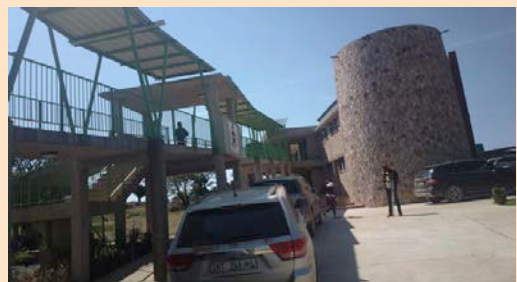
The school's administration block.
