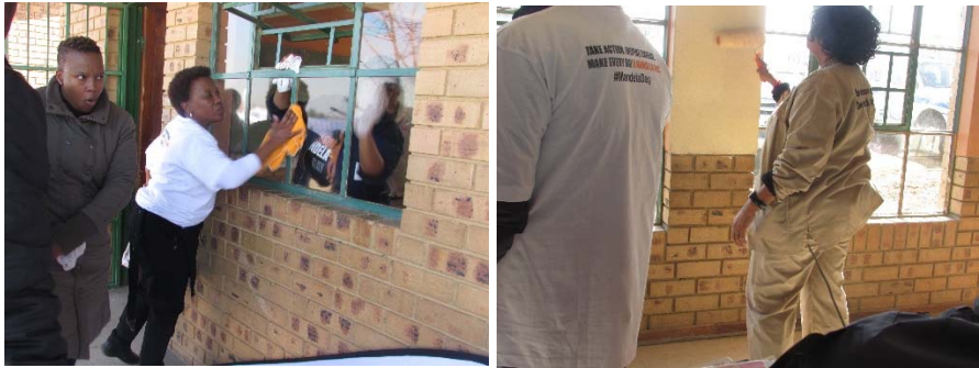
Sedibeng Employees Ms Tshwanelo Mokwari, Puleng Motloane, MMC Raikane cleaning and painting classrooms at Efford Primary School on Mandela Day
