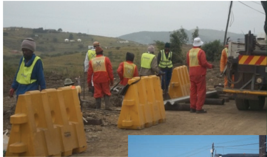
Tombo community members working on the project.
