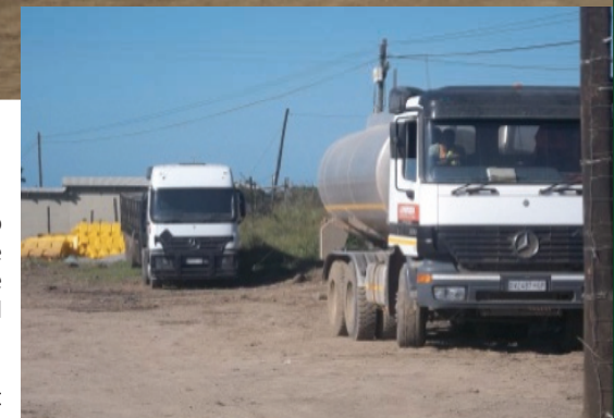
Construction site for the R61 Road revitalisation project.
