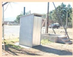
One of the complete erected ventilated improved pit toilets produced at the factory
