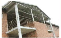
Part of the roof of the first-floor balcony falling apart.
